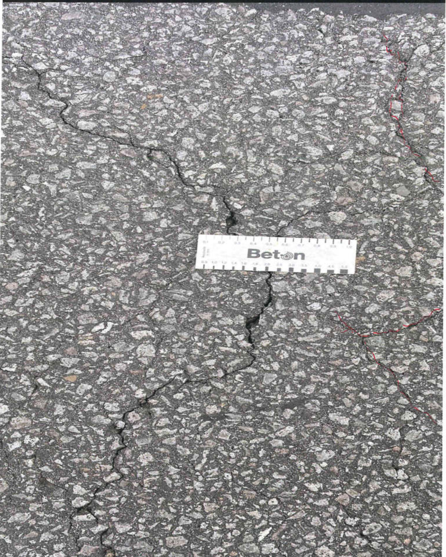
Schadbild A 20, AS NBG Nord - AS NBG Ost, beide Rifa Voruntersuchung km 251,172 - km 262,391
